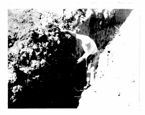
8. Trench excacated through U.S. slope Sta. 3+00<sup>+</sup>. Note delineated saturation line with very loose above and sl. consolidated below.
