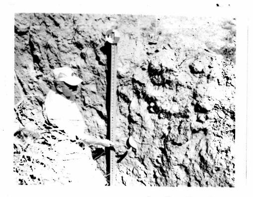
7. Profile of longitudinal crack Sta. 5+00<sup>+</sup>. Depth approx. 3'-0". Length 40'.
