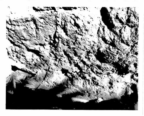
4. Foundation trench through failure section. Note contact of cutoff, gravel layer, and lake bed sediments.
