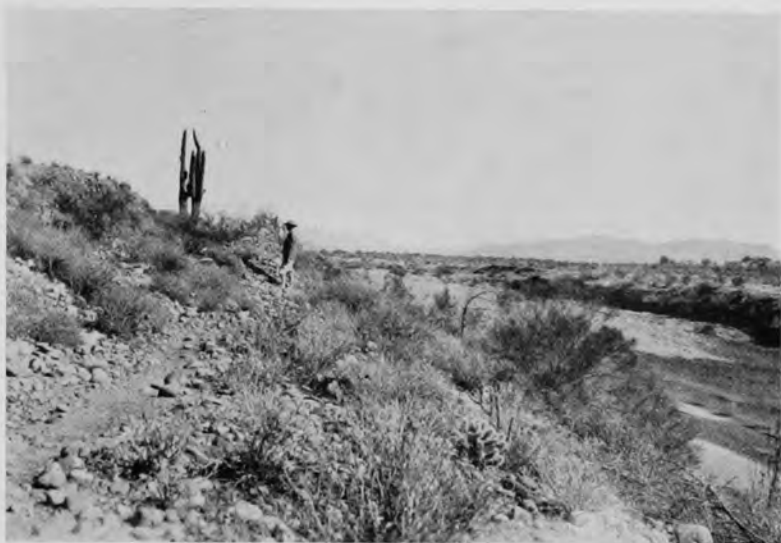
FIG. 140.—A partially destroyed ancient Indian canal west of Granite Reef dam, lying 25 feet above the present bed of Salt River. (Photograph by Judd.)
