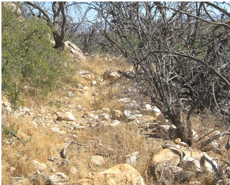
Figure 3. Looking down canal at the narrow, nearly completely filled Robinson Canal as it routes along the steep mesa side on its way to fields on Robinson Flat. Note the canal coursing upslope illusion.
