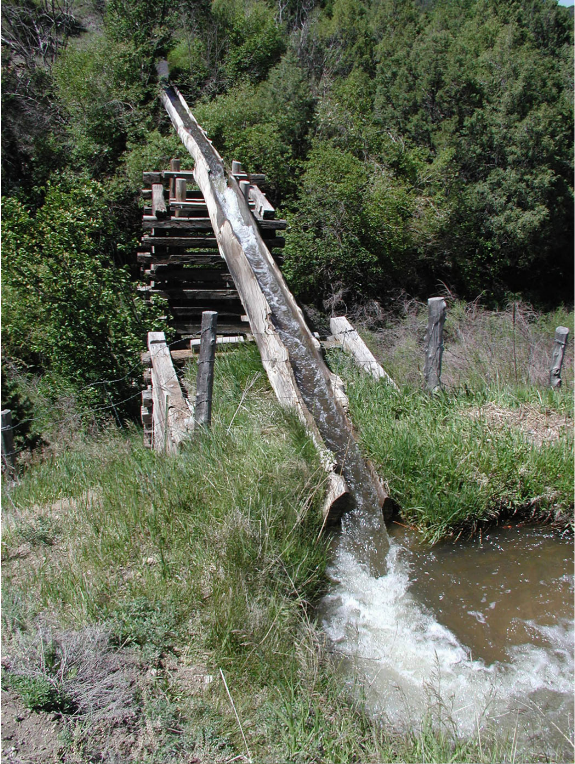
Figure 23. Another view of the Trampas, New Mexico canoa, looking south. Two long logs have been cut to form U-shaped channels, and then partially overlapped to span the arroyo.
