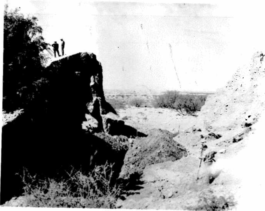
1. Looking northwest through washout - Sta. 2+50 \pm .
