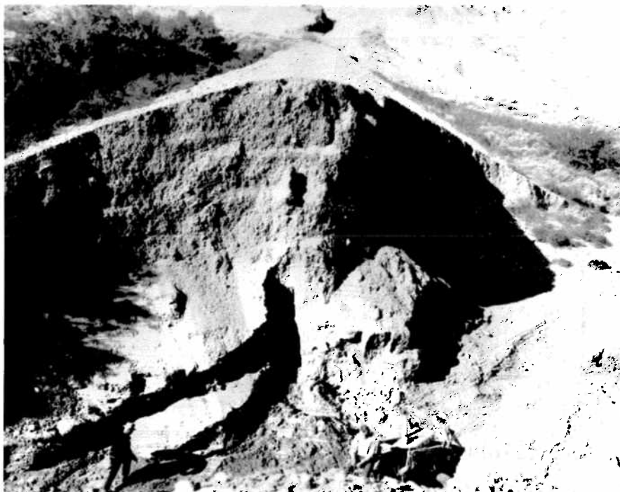
2. Looking west facing failure section Sta. 2+00 \pm .
