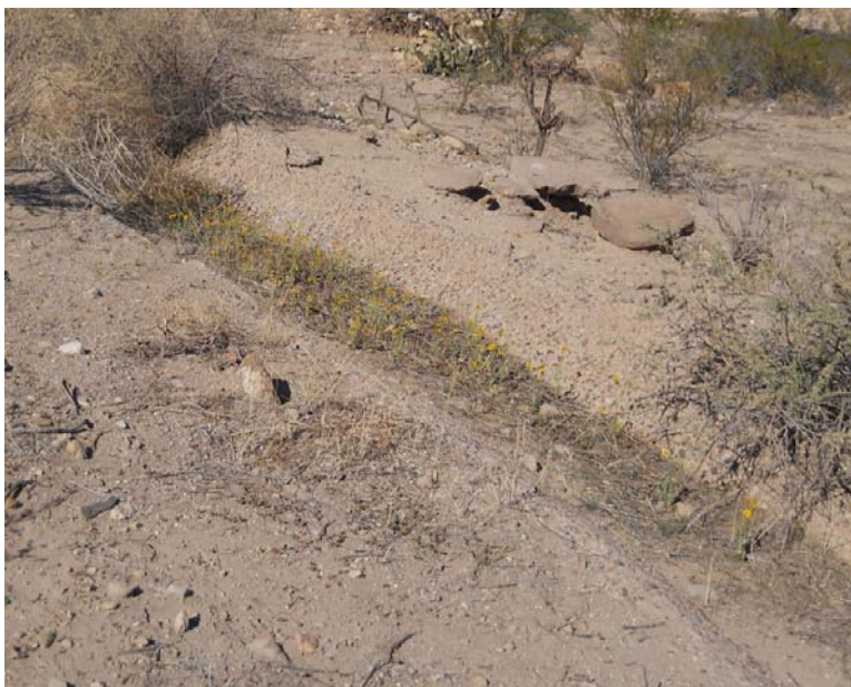
TRANQ2 – A closeup of the historically reworked coarse aggregate canal lining that resembles similar rework on the Marijilda Canal. The view is to the north at 32.76485 -109.72952 .
