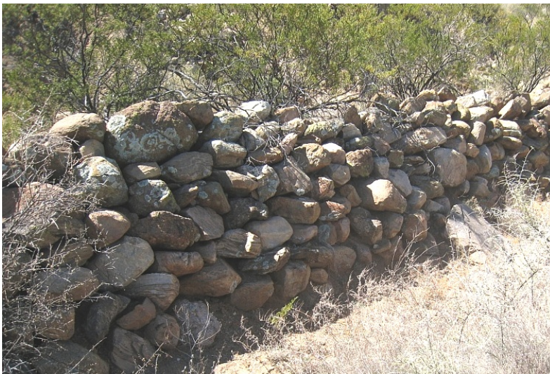
FRYE106 – This seems to be the highest wall in the entire canal system and remains quite enigmatic. The rocks appear to be carefully size sorted. View is to the east near 32.76752 -109.79273 .
