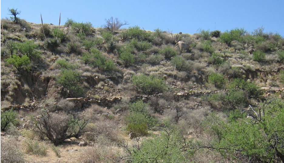
FRYE100 – On approach, this portion of the Lower Frye Construct appears very similar to other hanging canals in the system. Especially 32.79950 -109.96378 on the Sand Canal . View is to the east from 32.76816 -109.79196
