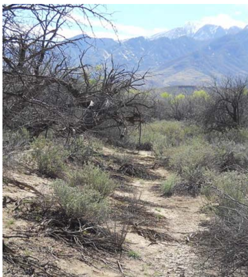
CLUFFNW2 – The second historic rebuild created a huge water channel whose size suggests Gradall class machinery and high construction energy inefficiency. Portions are unusually single walled. View is south at N 32.82625 W 109.84596 .
