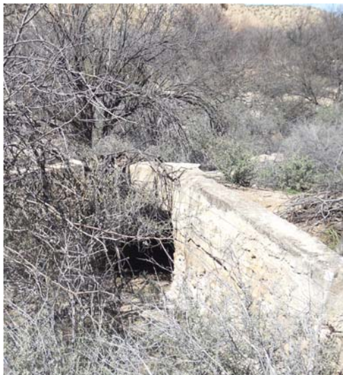
CLLUFFNW1 – One of several Y-Weir concrete structures from the second historical rebuild of the Cluff NW canals. This one was apparently part of a wash crossing inverted siphon. Viewed northwest from N 32.82647 W 109.84590 .
