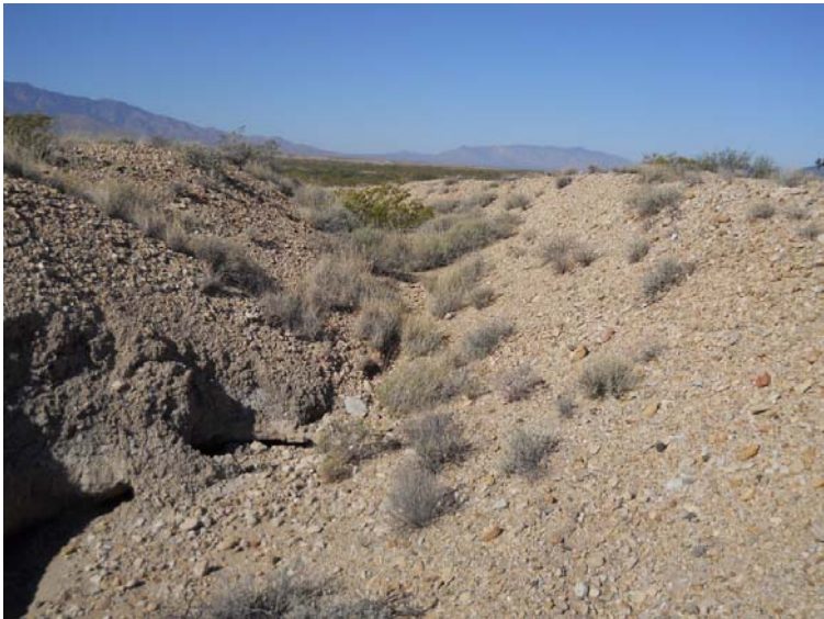
CULEBRA2 – There appears to be some flood damage just before the start of the major Culebra Cut. Three included canal constructs are the Culebra, the aquaduct, and the HS canal. The view is to the west at 32.83569 -109.79794
