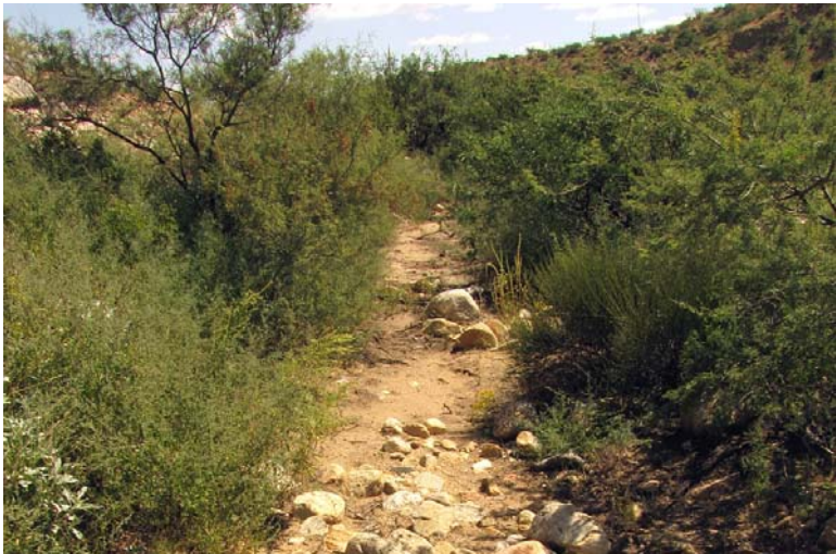
ALLENO – Just after its rather elaborate takein structure, the Allen Canal changes direction and begins a "climb" to the historic Hawk Hollow tank.. The view is to the north at 32.78252 - 109.83453
